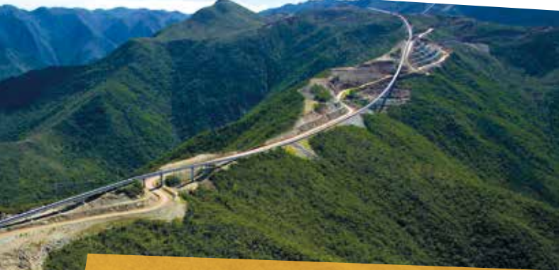
带式输送机 | Belt Conveyor
